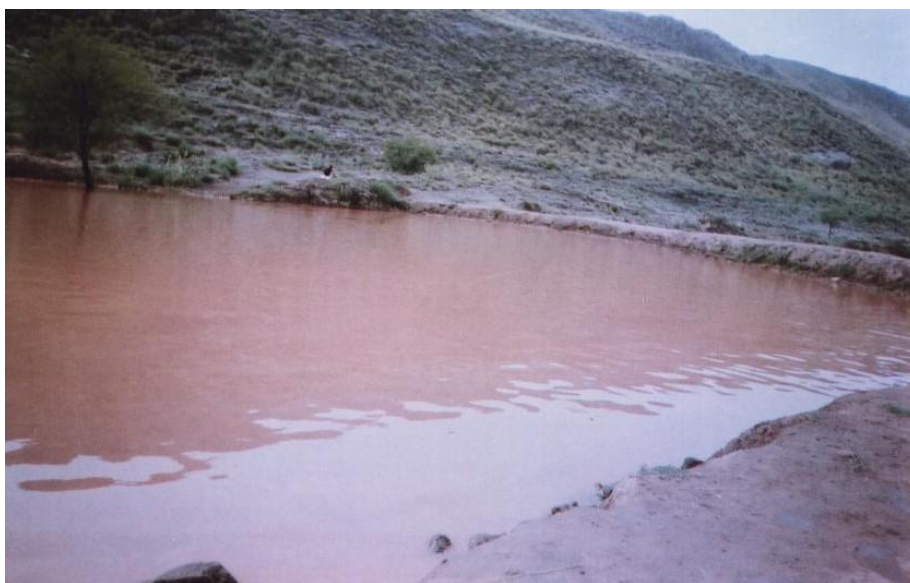
Plate 3: Check Dam Karak (Photograph from M.Yasin SWCO Karak)
