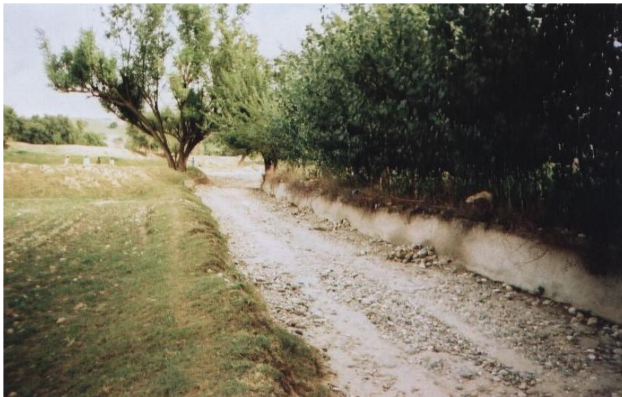
Plate 2: Protective Bund in Ghundi Mir Khan Khel (Photograph from M.Yasin SWCO Karak)
