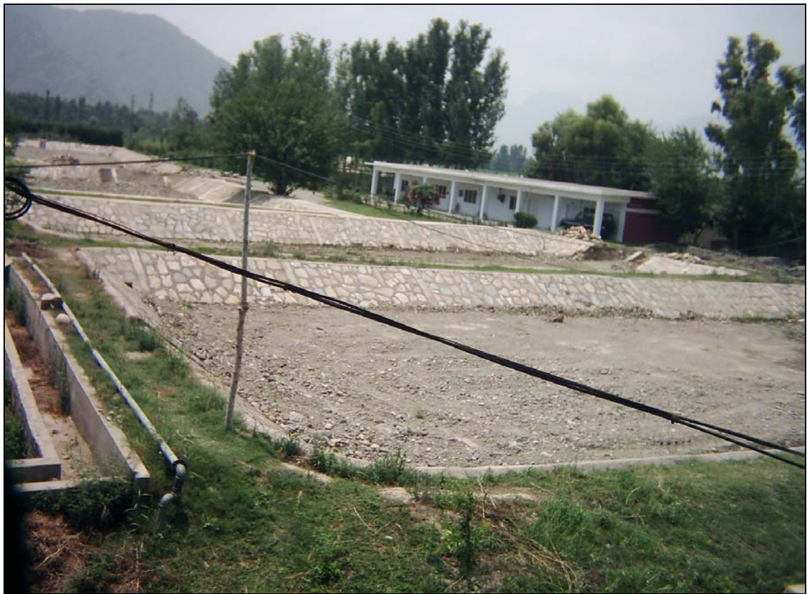
Pic. F. 40:- Fish Pond Under Construction, Which Will Receive Mashair Fish (One of the Endanger Species of Malakand Division) From Pond Shown in Picture 67. After the Construction of these Ponds it is hoped that Aquaculture will start in Dir, Swat and Malakand Still a Long Way to go. Picture Taken in Fisheries Office Situated Opposite of Chakdara Fishing Hut.
