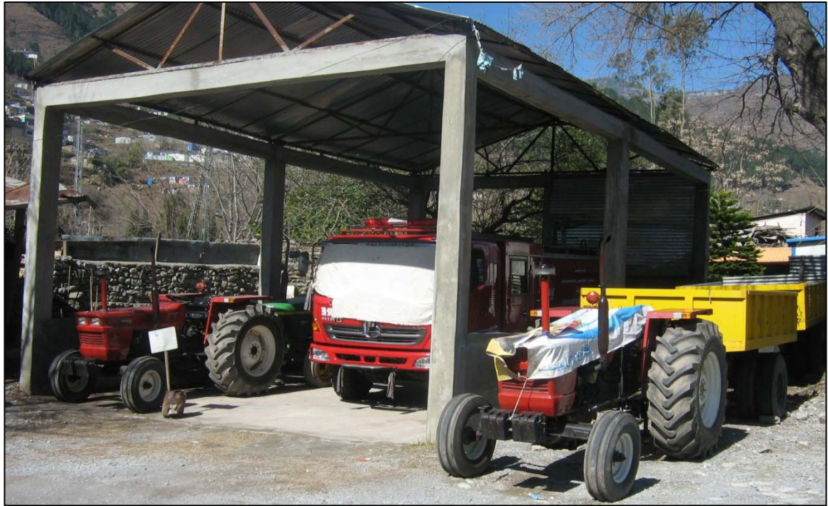
Figure 4.10 TMA Office, Balakot
