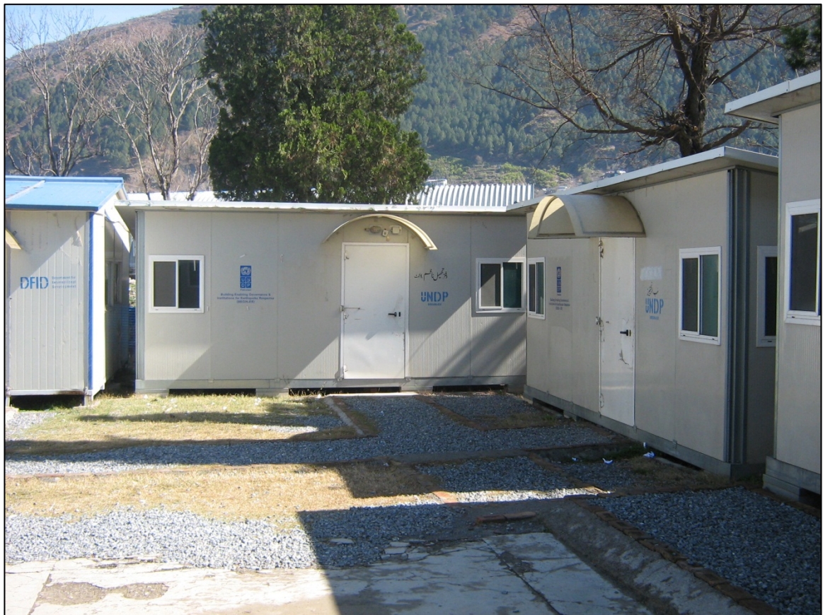
Figure 4.11 TMA Office, Balakot
