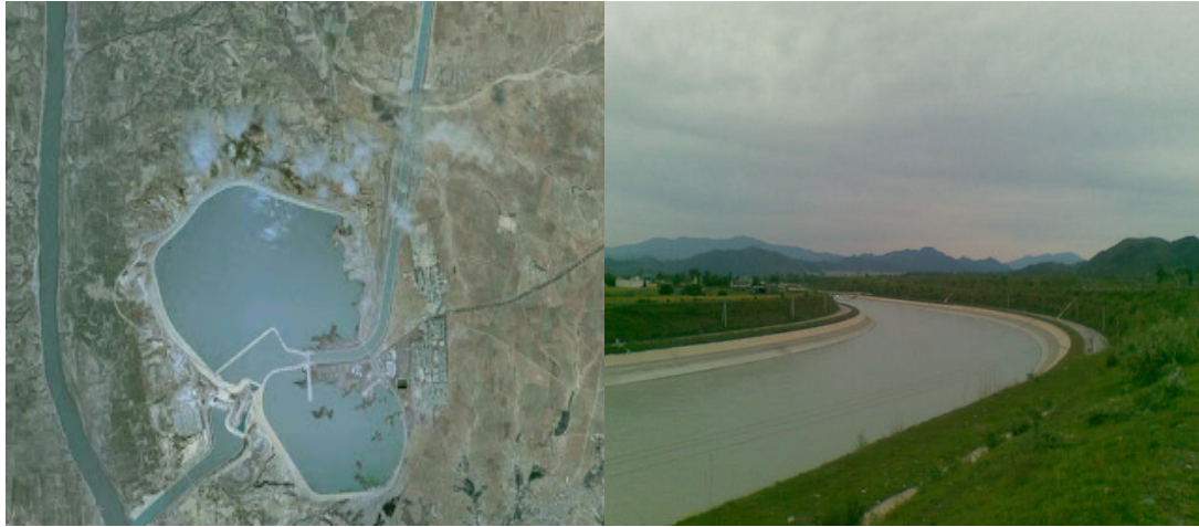
Figure-7.2: Ghazi Barotha dam and bypass canal
