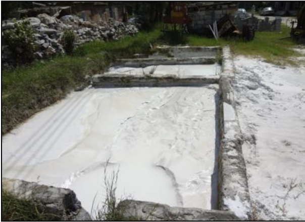
Photo 11: Settling tanks filled from Slurry wastes
