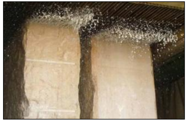
Photo 6: Gangsaws Cutting of Marble blocks
