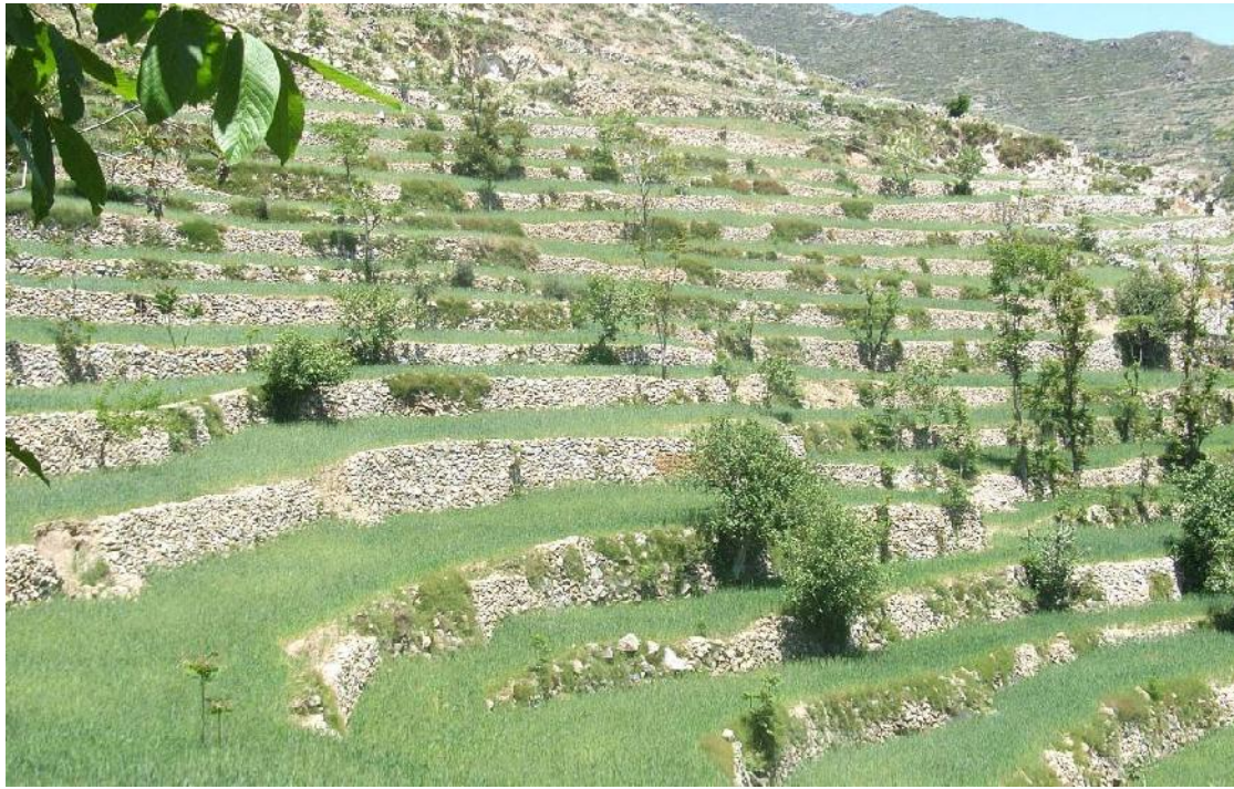
Fig 4.7 Rain-Fed Cultivated Terraces on Hill Slopes around the Village
