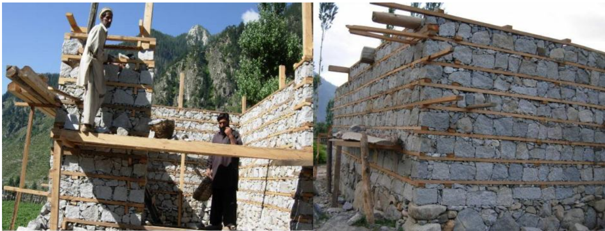
Fig 5.8 Present use of Timber Wood in Construction of Houses
