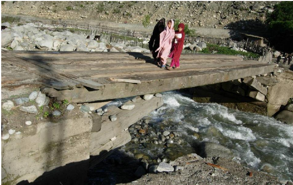
Fig 5.10 Locally Constructed Wooden Bridge in Thal Village in Thal
