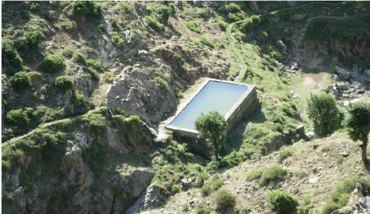
Fig 4.6 Water Storage Reservoir Constructed by the Community
