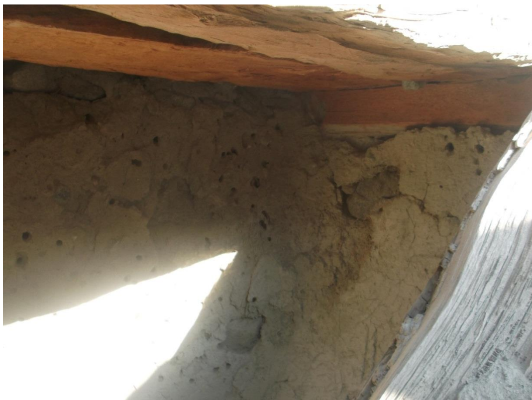
Plate CXXXVII: Gurunjur—covered roof over the grave no. 2.
