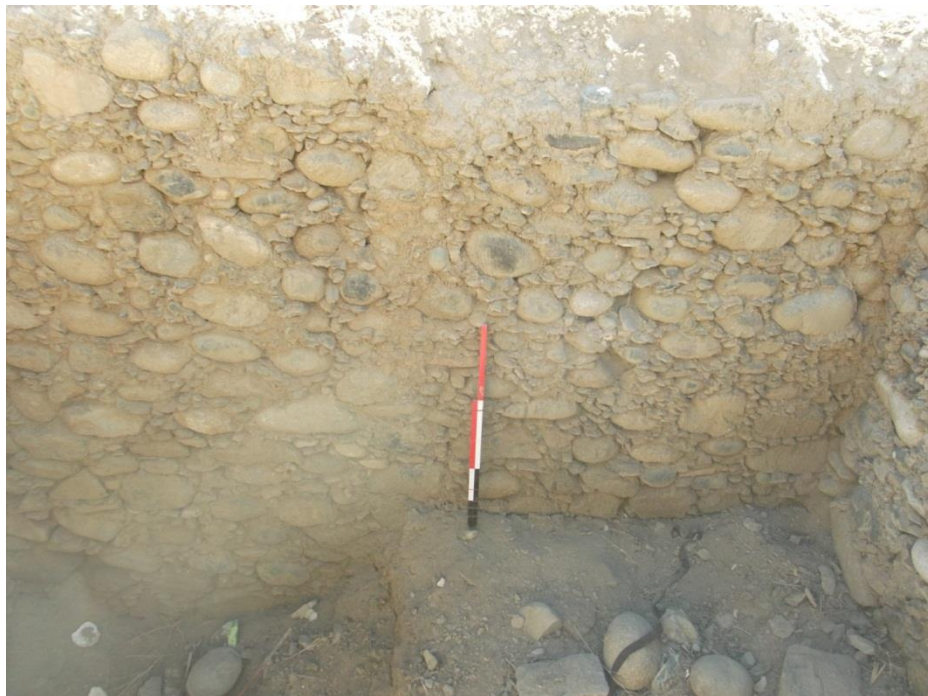
Plate CX: Sumal—details of interior exposed structures, presenting the masonry of southern side wall's interior.
