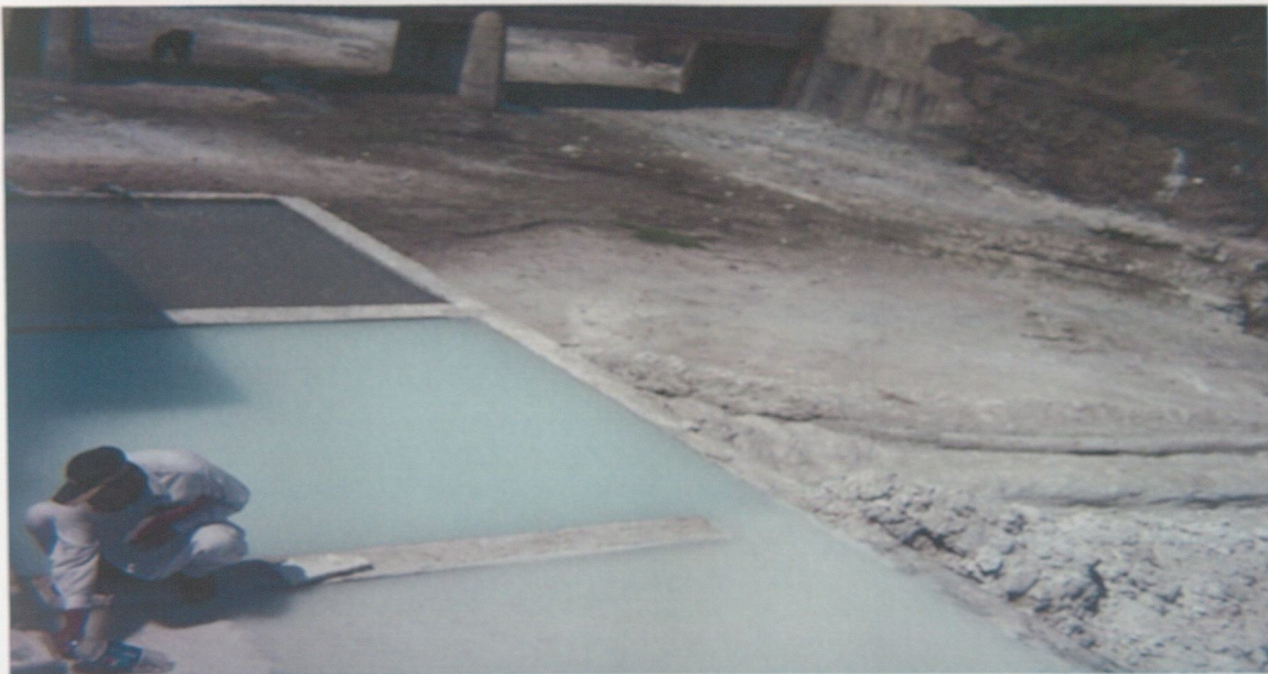
Effluent drain of Shalman Marble in HIE Peshawar Sample # 3
