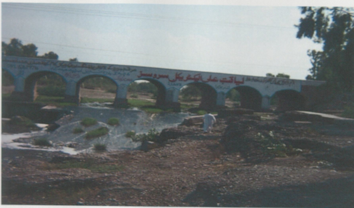
Main effluent drain near board bridge where B.Naran "Khwar" meet with it sample # 23
