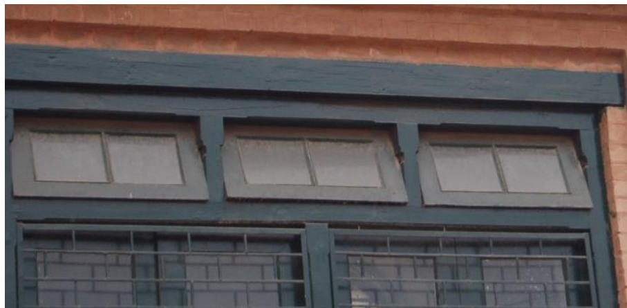
Plate 80: Islamia College Peshawar, rectangular shaped ventilator in class room.
