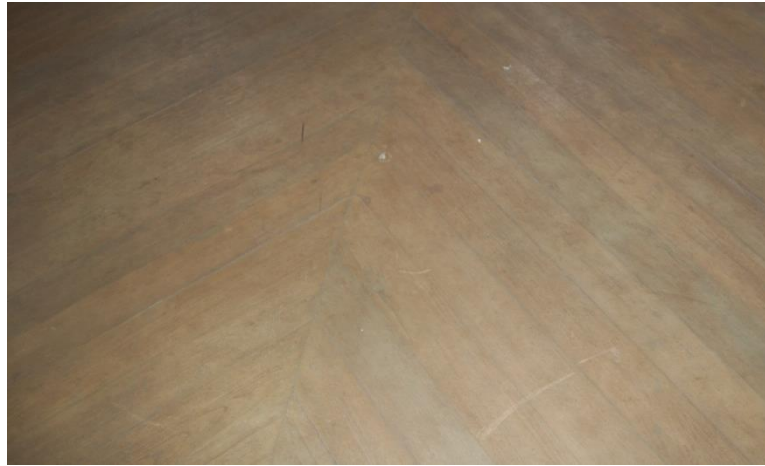
Plate 29: Islamia College Peshawar, wooden floors in Roos Keppel Hall.
