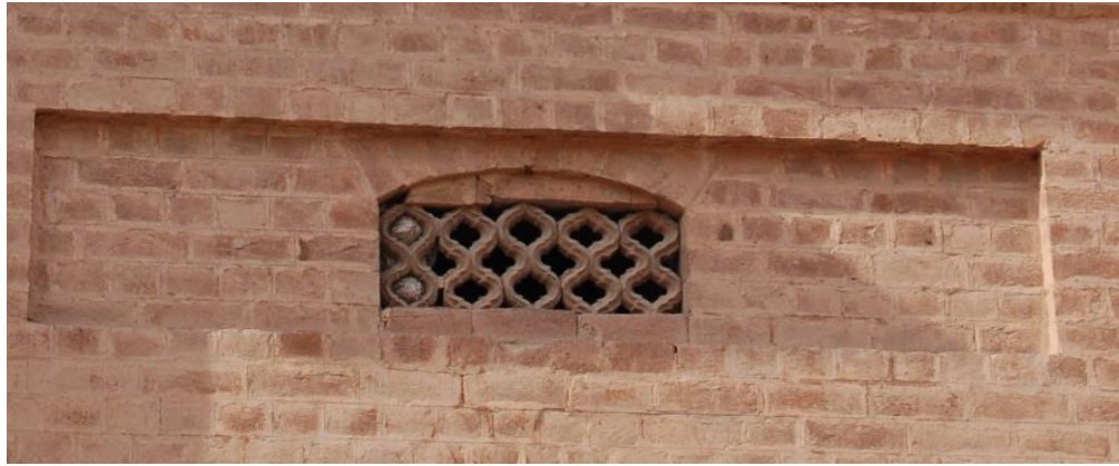
Plate 83: Islamia College Peshawar, fret work ventilator.
