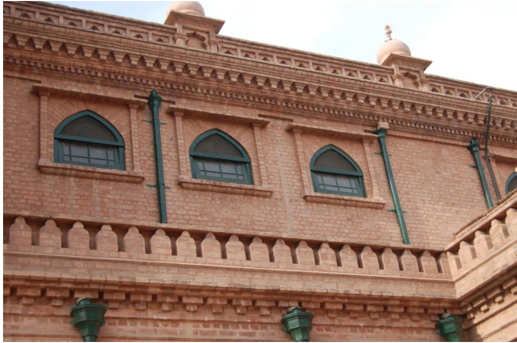
Plate 56: Islamia College Peshawar, brick work of exterior wall.
