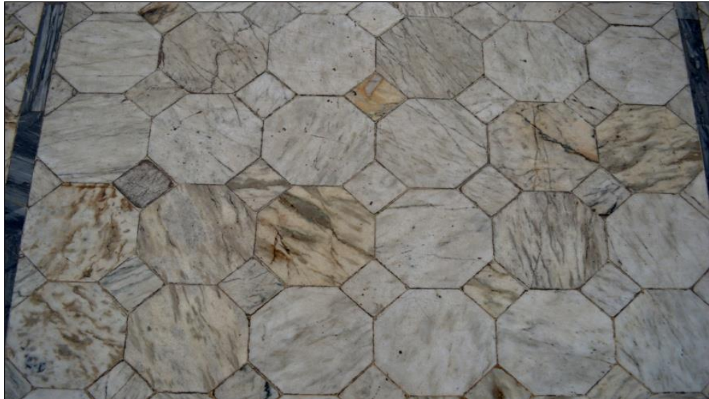
Plate 65: Islamia College Peshawar, floors in hostel.
