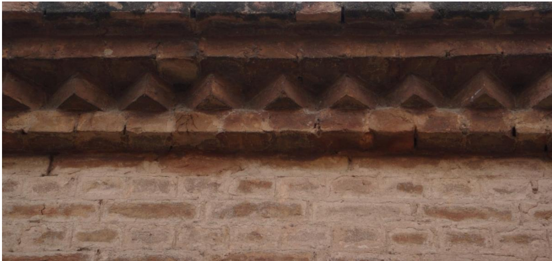
Plate 130: Islamia College Peshawar, saw tooth brick pattern.
