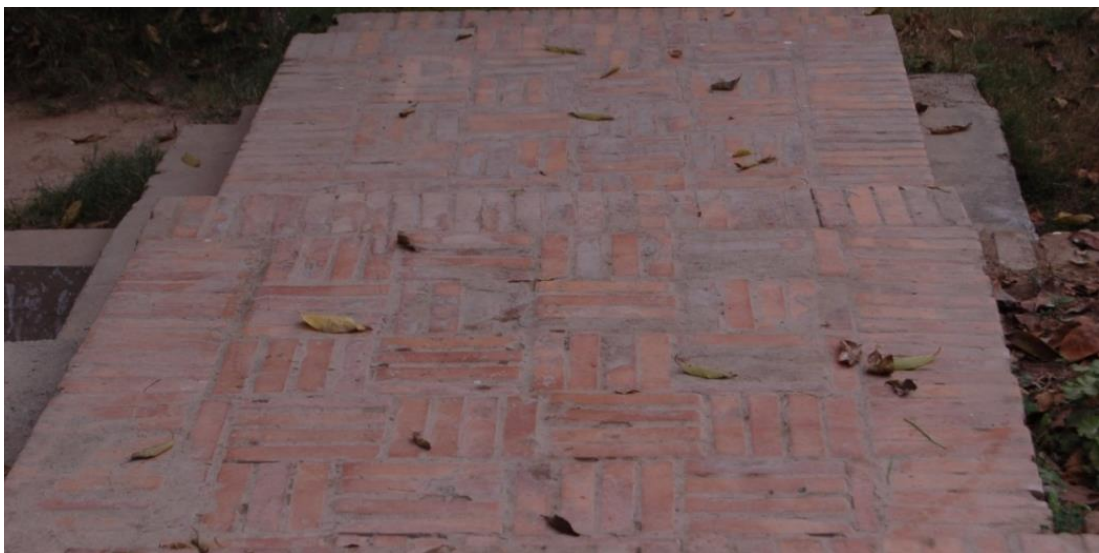
Plate 135a: Islamia College Peshawar, basket weave brick laying on floor.
