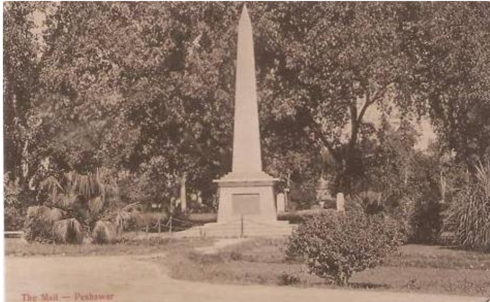
Plate 6: Peshawar, a general view of Mackenson Memorial.
