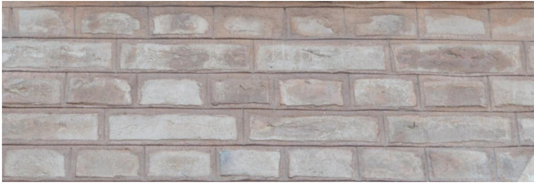
Plate 131: Islamia College Peshawar, header and stretcher brick laying.
