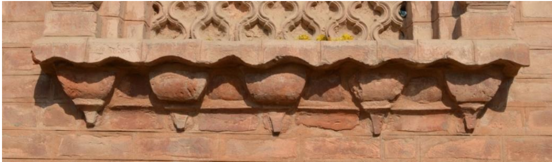
Plate 134: Islamia College Peshawar, cut and dressed brick shapes used in decorative windows.
