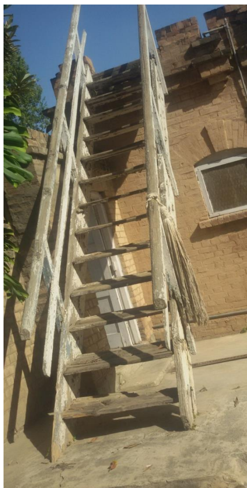
Plate 37: Islamia College Peshawar, wooden stair case in residential area.
