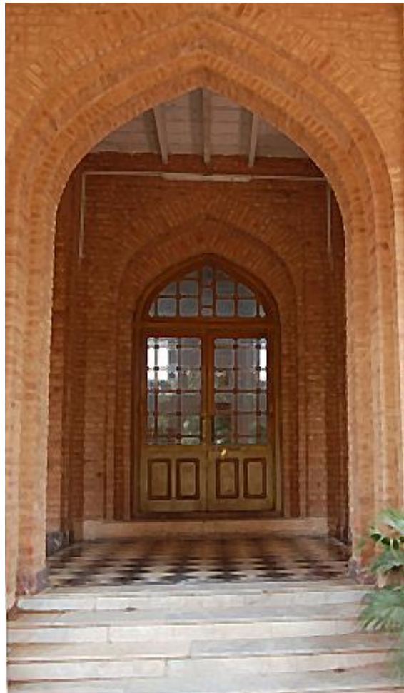
Plate 24: Islamia College Peshawar, entrance of Roos Keppel Hall.
