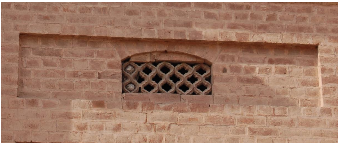
Plate 123: Islamia College Peshawar, fret work ventilator in sunk panel.
