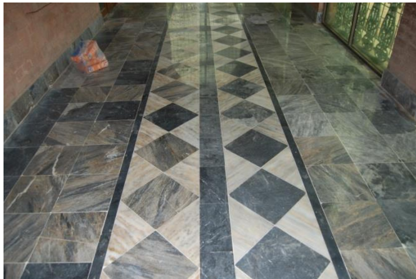
Plate 60: Islamia College Peshawar, verandah floors.
