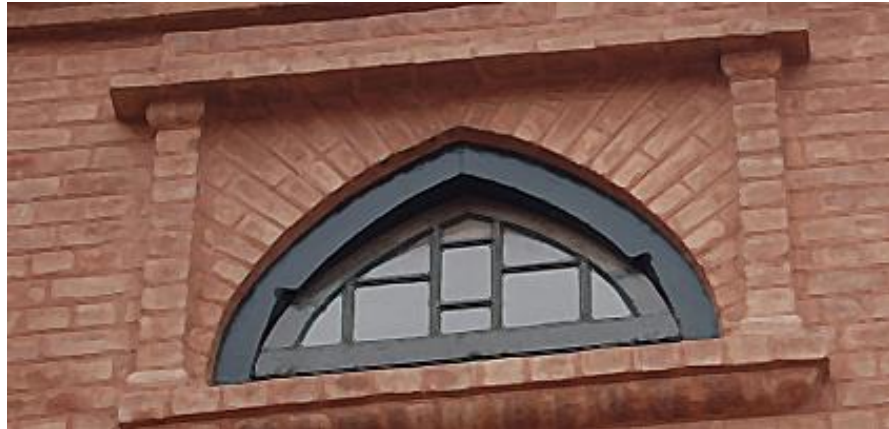
Plate 79: Islamia College Peshawar, arch-shaped in D shaped ventilator. (Outer View)
