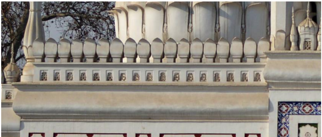
Plate 115b: Islamia College Peshawar, parapet in Mosque (Second Step).
