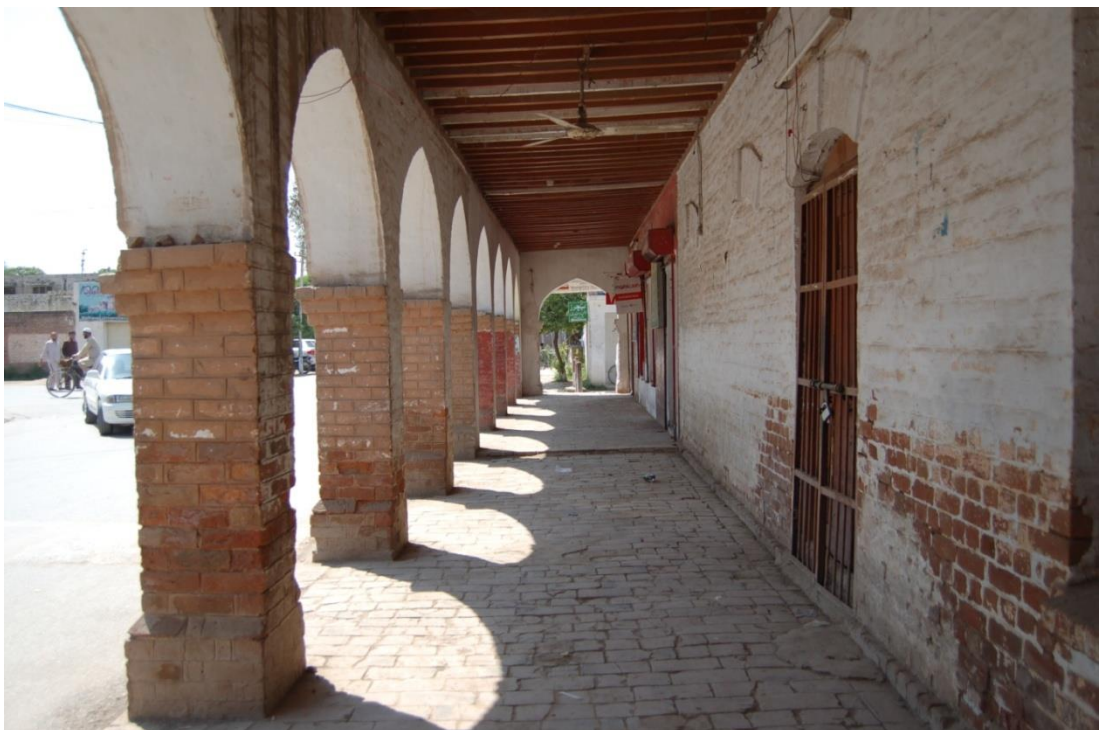
Plate 54: Islamia College Peshawar, verandah in Khyber House.
