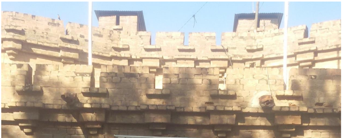
Plate 114: Islamia College Peshawar, panel style parapet wall in residential area.
