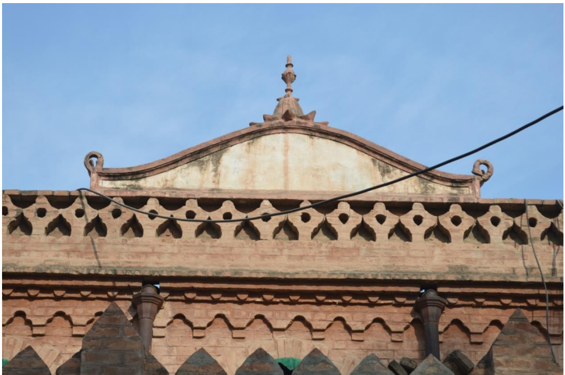
Plate 49: Islamia College Peshawar, running merlons, parapet and insignia slab.
