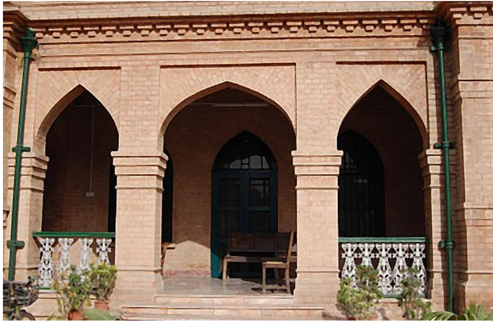
Plate 86: Islamia College Peshawar, square-shaped columns.
