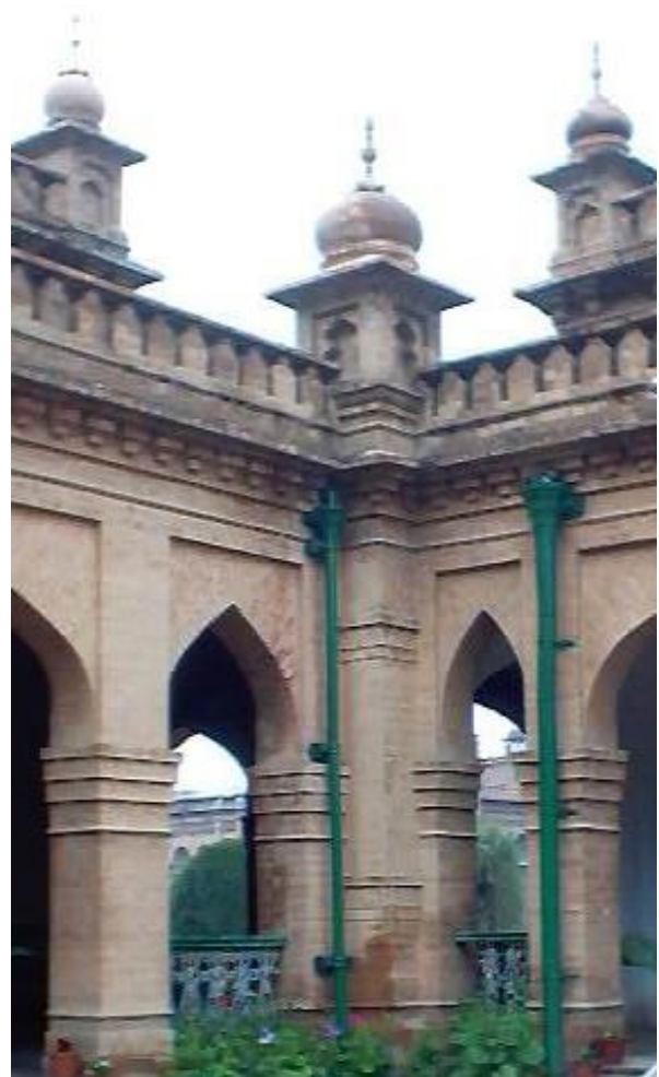
Plate 95: Islamia College Peshawar, dome with cut brick work.
