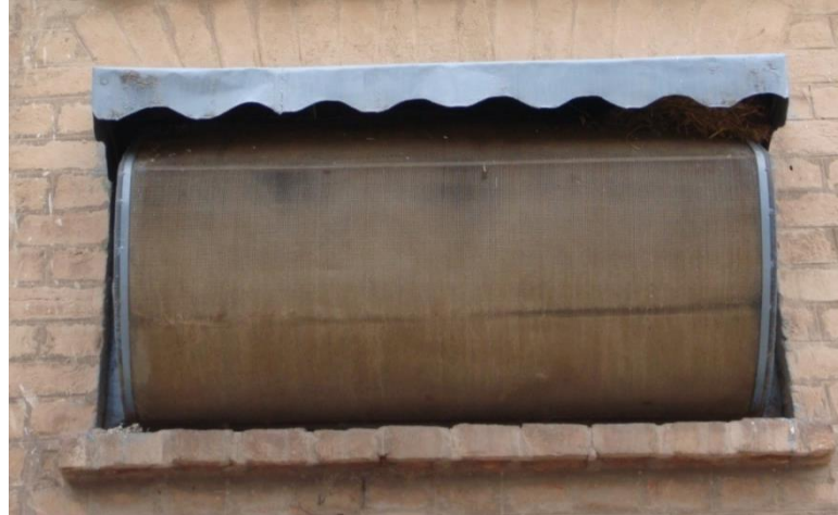
Plate 81: Islamia College Peshawar, rectangular shaped ventilator covered with wire gauze.
