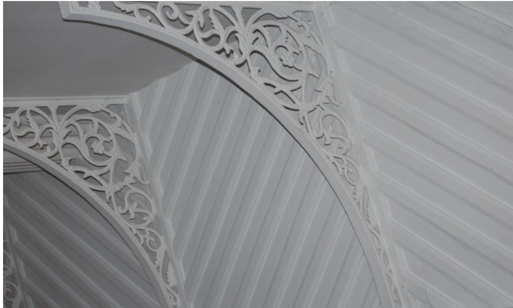
Plate 32: Islamia College Peshawar, brackets for the support of gallery in Roos Keppel Hall.
