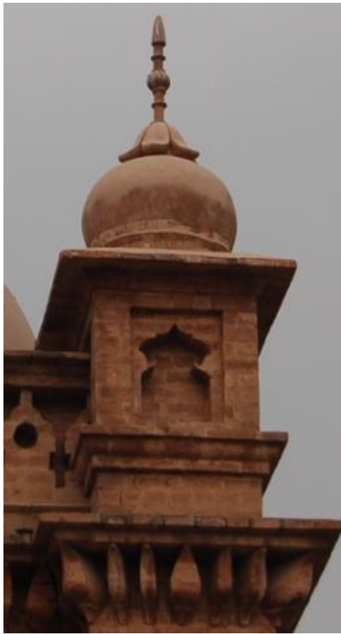
Plate 94: Islamia College Peshawar, chatrus embellished with arches and brick work.
