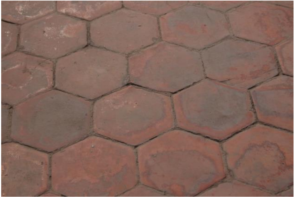
Plate 63: Islamia College Peshawar, hexagonal floor tiles.
