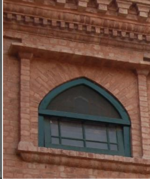
Plate 78b: Islamia College Peshawar, ventilator in Roos Keppel Hall. (Outer View)
