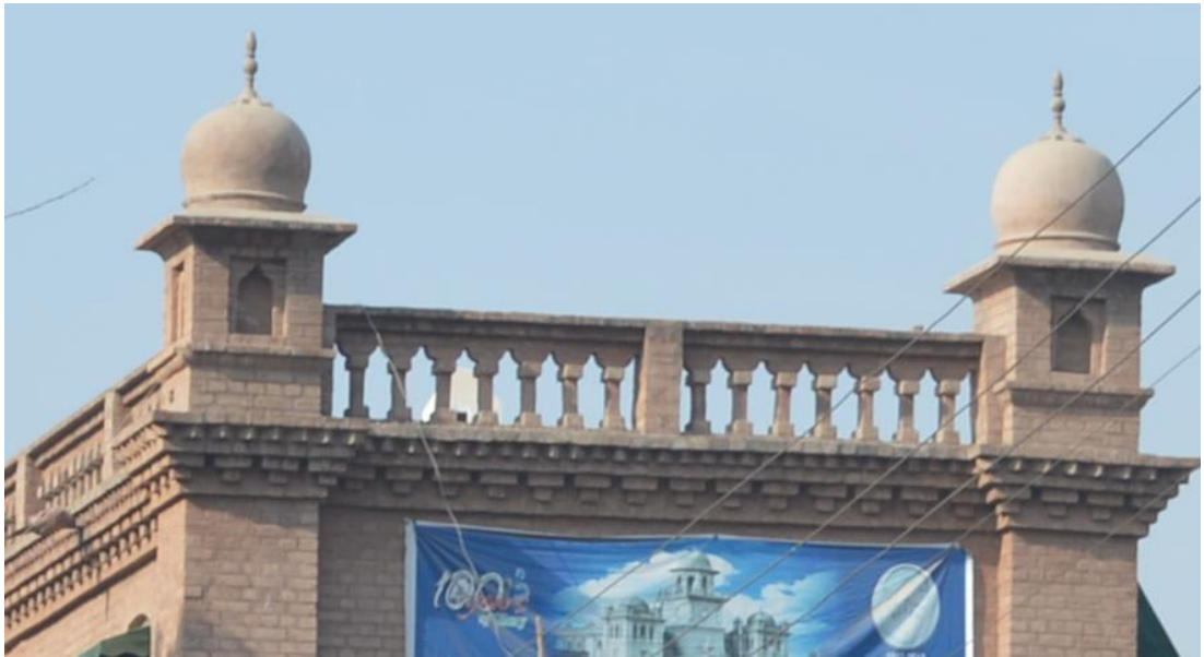
Plate 113: Islamia College Peshawar, perforated style parapets.
